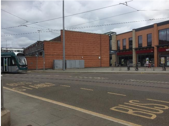
Site from south
