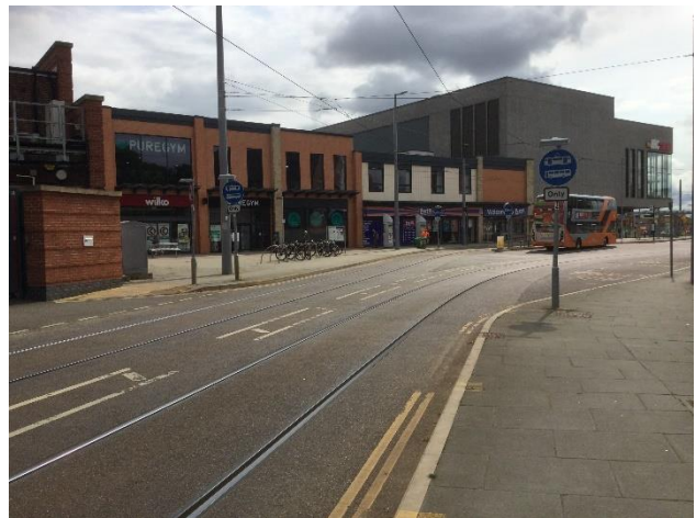
Site from west (with new cinema to RHS)
